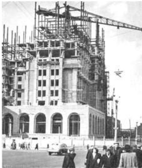
The construction of new Moscow
